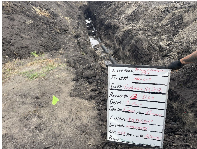
Facing west at MP 31.63, completed a drain tile repair
