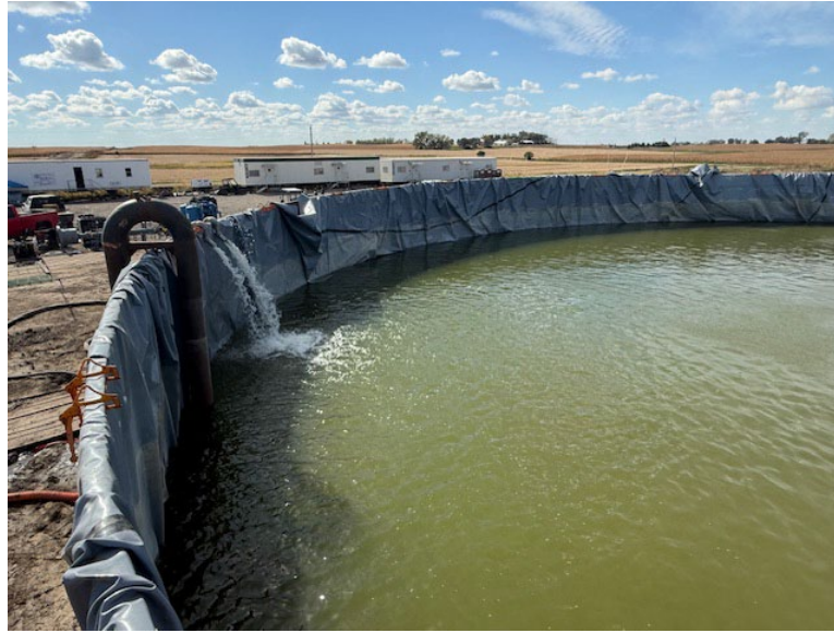
Facing southwest at MP 34.2, dewatering hydrostatic test water to lake tank
