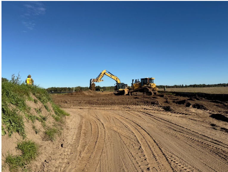
Facing north at MP 1.52, view of Otis commencing restoration of the topsoil
