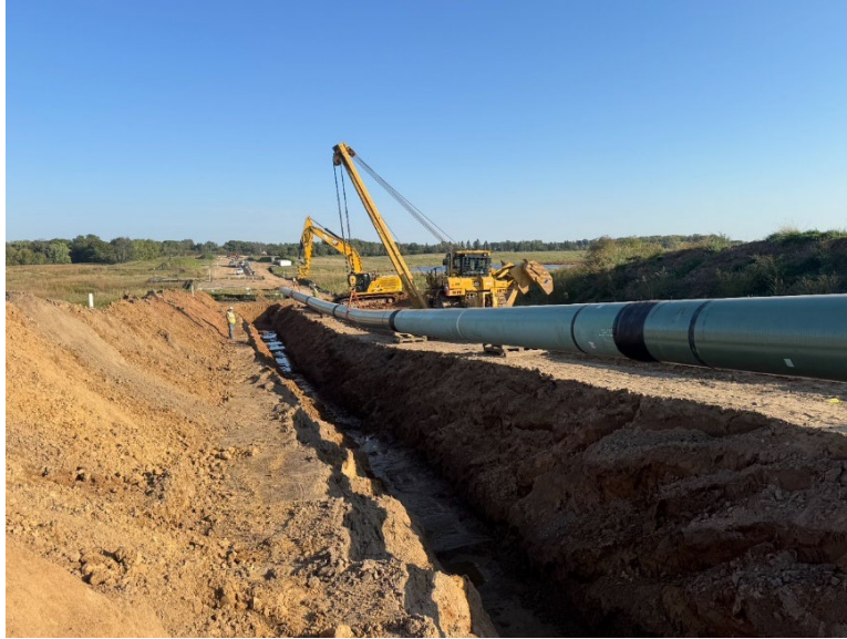
Facing north at MP 1.45, view of Otis lowering-in pipe
