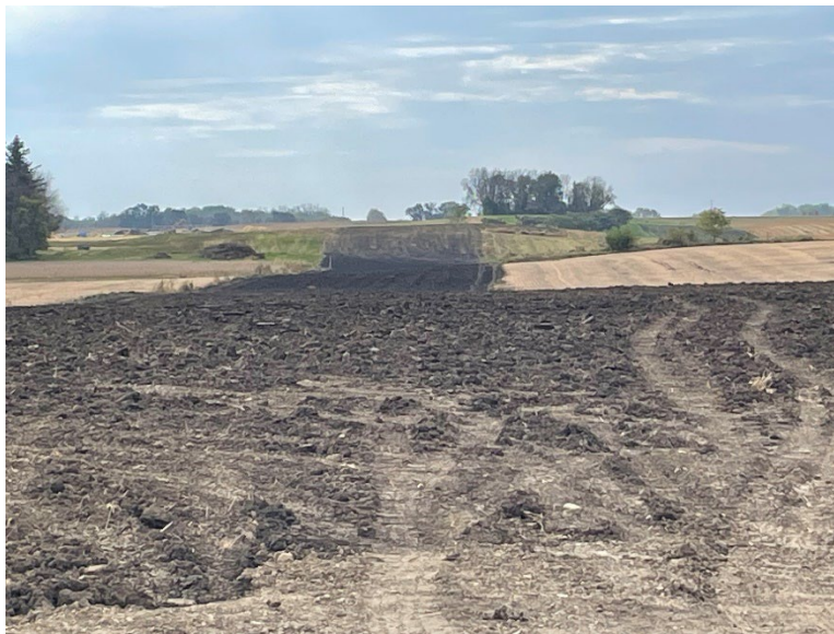
Facing south at MP 31.95, topsoil brought to grade south of 140th Street
