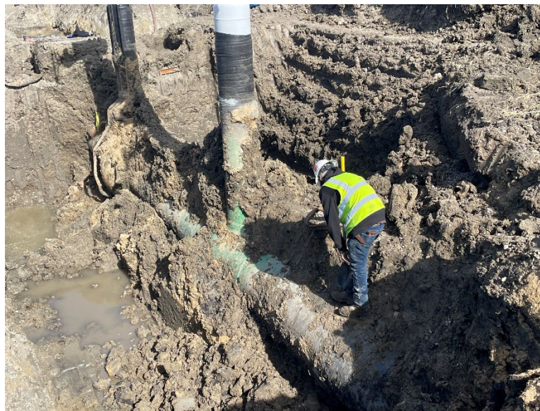
Facing north at MP 31.2, K&K hand excavating near valve setting
