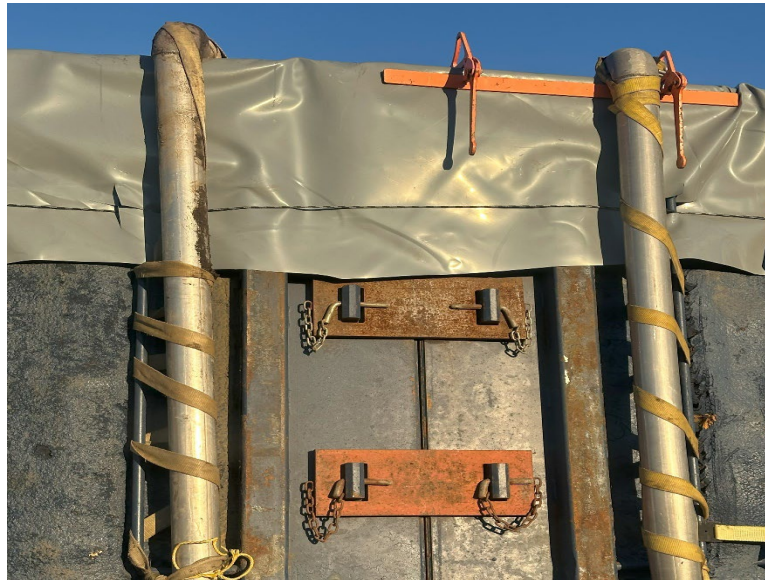
Facing northwest at Milepost 34.2, north of 165th Street, contractor has lashed discharge piping to lake tank
