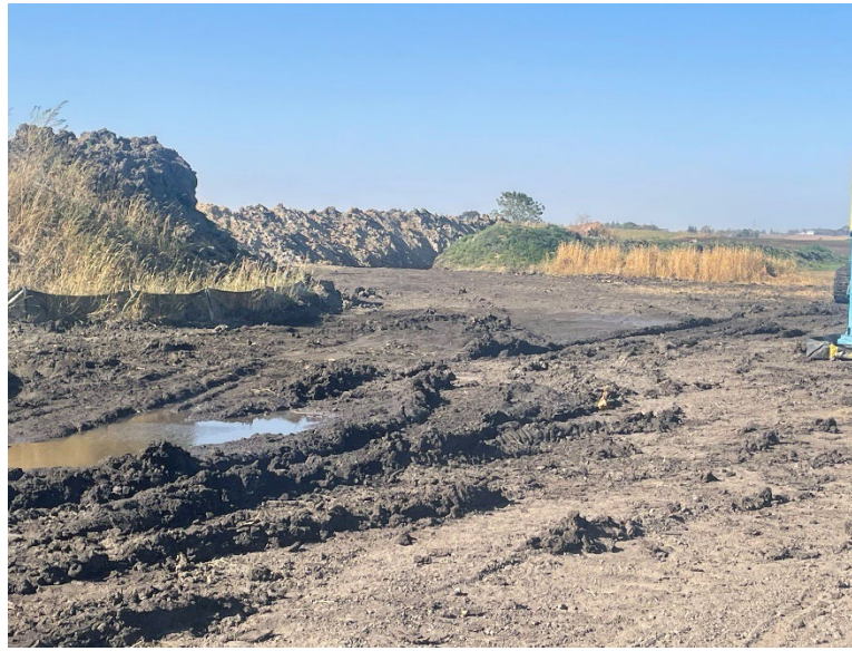
Facing north at MP 31.2, north of County Highway 9/135th Street, majority of the water has infiltrated into the ground and the frac tank relocated
