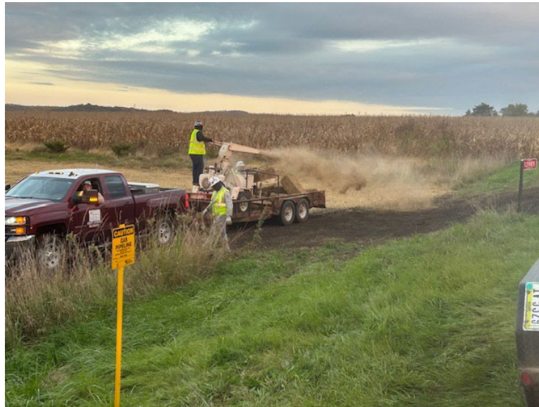
Facing north on west side County Road B, K&K mulching row
