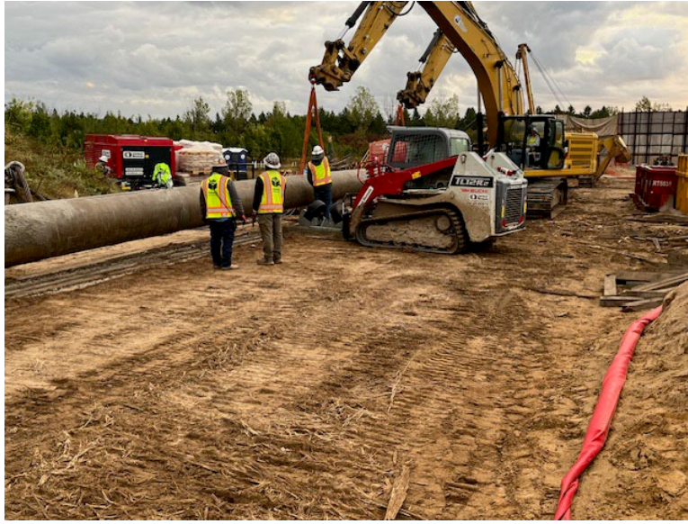
Facing east HDD P4-5 bore pipe extraction was completed
