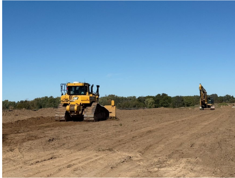
Facing north at MP 1.52, view of Otis continuing restoration of the topsoil
