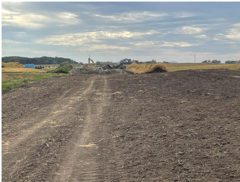
Facing south at MP 31.45, topsoil brought to grade south of 140th Street
