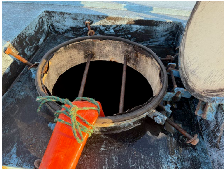
Hose that came out of frac tank has been secured to the hatch
