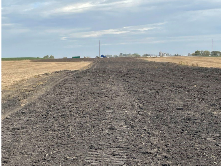
Facing north at MP 31.7, topsoil brought to grade south of 140th Street
