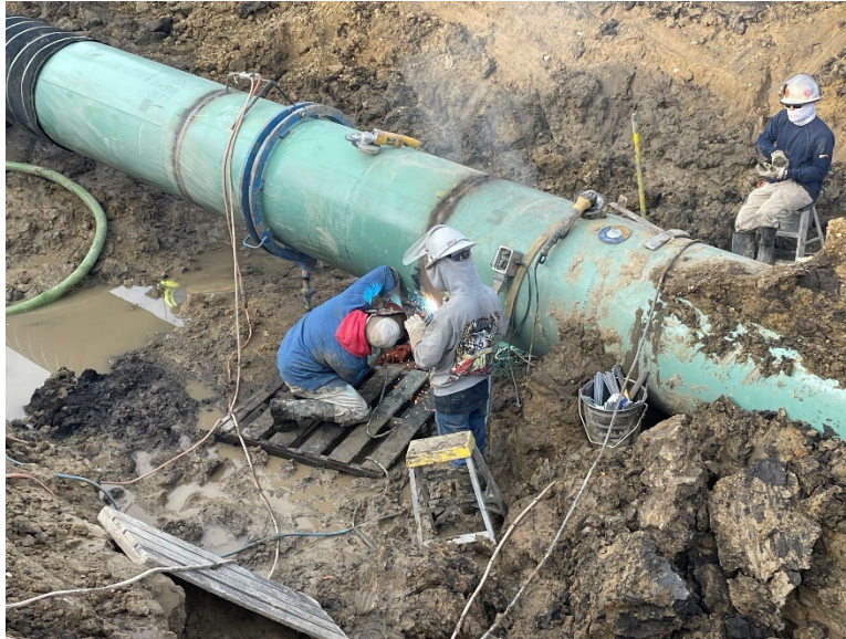
Facing southwest at MP 33.7, K&K completing a mainline trench tie-in weld
