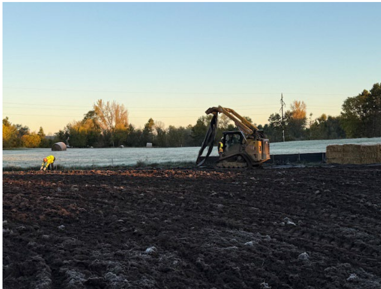
Facing west near MP 2.14, ECD removal ongoing
