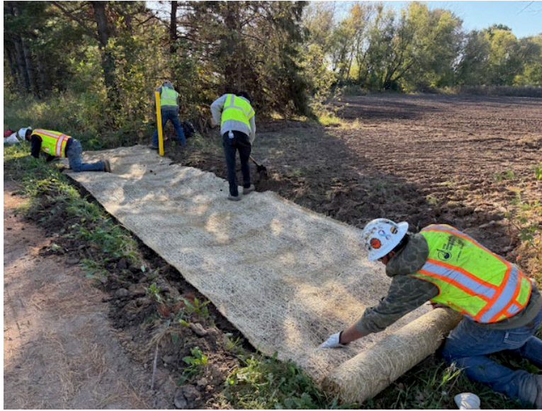
Facing north near MP 3.4, road approach restoration commenced
