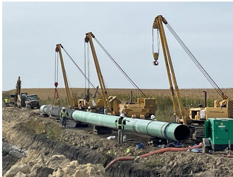
Facing southwest at MP 33.7, K&K lowering-in a four-joint section of mainline pipe south of 165th Street
