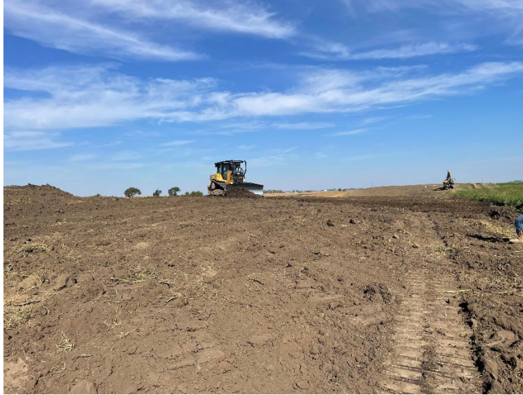
Facing south at MP 31.5, K&K restoring topsoil to grade south of County Road 9/135th Street
