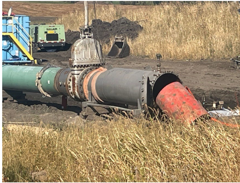
Facing northeast at MP 31.2, foam pig that will be used to remove remaining hydrostatic test water from mainline
