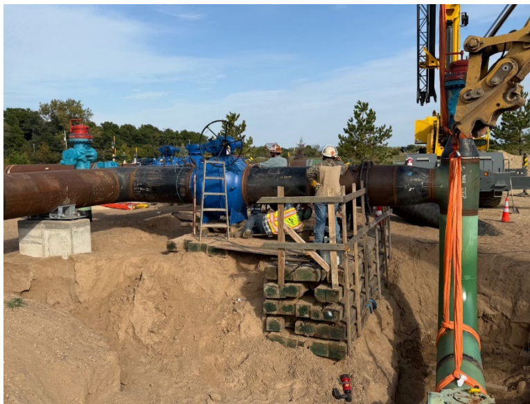
Facing east MP 0.01, view of Otis completing the last tie-in at the Hugo compressor station
