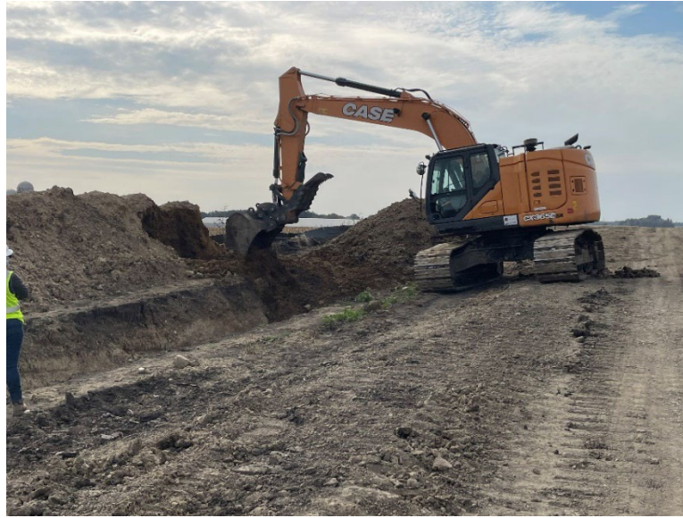
Facing southeast at MP 31.8, K&K backfilling trench north of 140th Street
