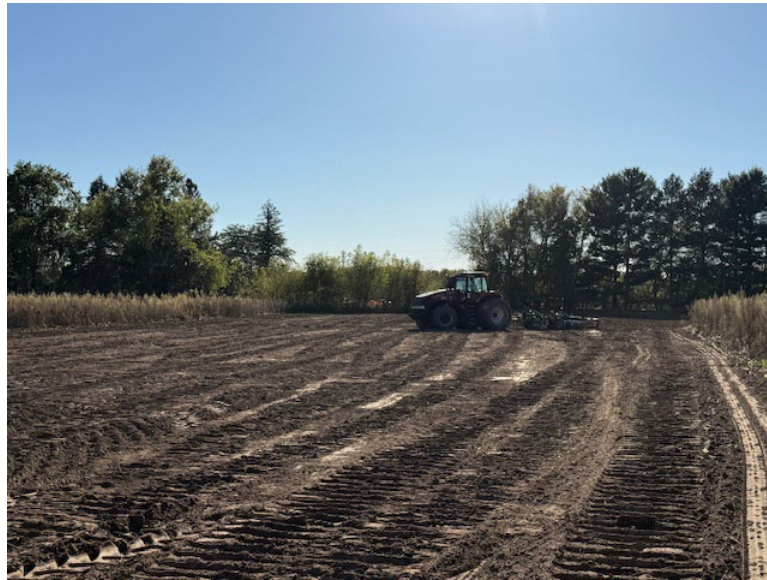
Facing east near MP 3.25, topsoil decompaction commenced
