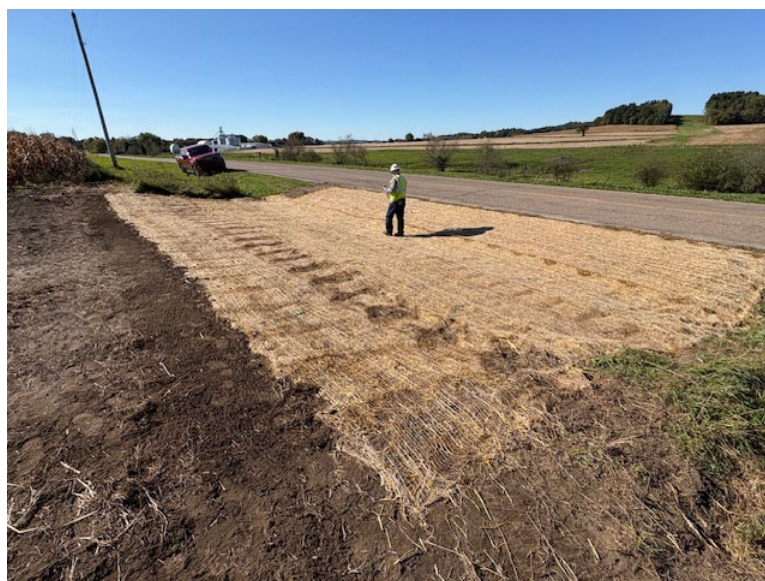
Facing south near MP 3.5, K&K installing ECBs at entrance to staging area
