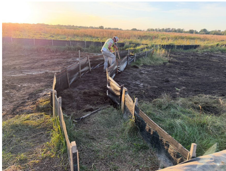
Facing west at MP 1.4, view of Otis reinstalling the redundant silt fence after completing wetland (FRM-W12) restoration
