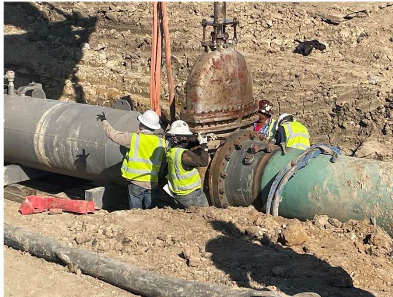
Facing northeast at MP 34.2, K&K installing launcher/receiver north of 165th Street
