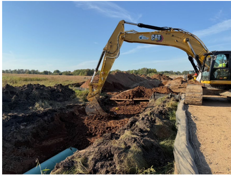
Facing north at MP 1.38, view of Otis backfilling the wetland (FRM-W13) from timber mats
