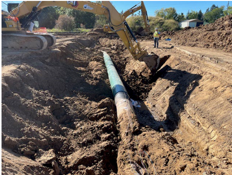
Facing east near MP 2.13, backfill ongoing
