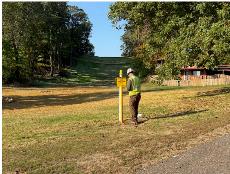
Facing west near MP 2.53, K&K installing pipeline markers
