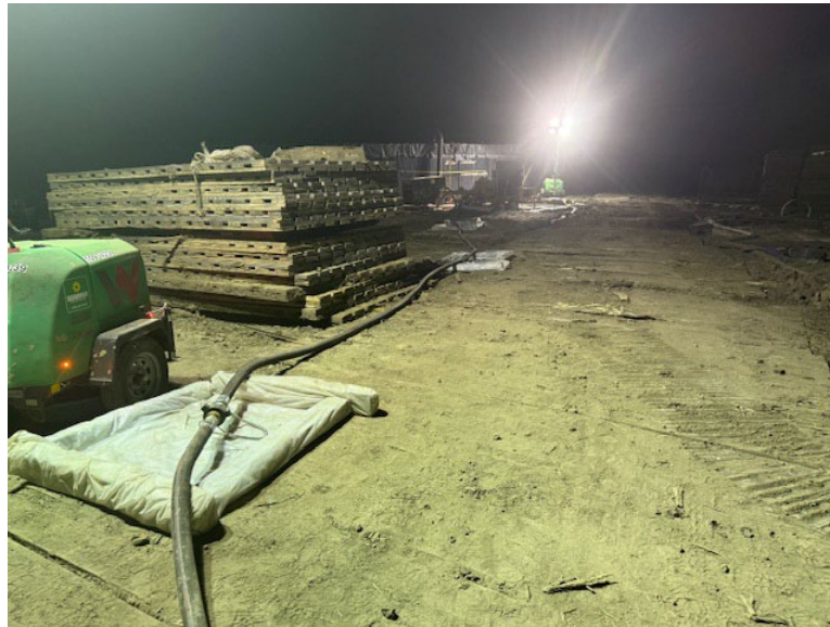
Facing north at MP 34.2, hydrostatic test in progress with secondary containment in place for dewatering line connection
