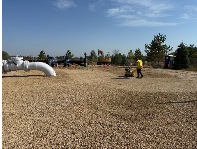
Facing east at MP 0.01, view of Otis backfilling with compaction in the Hugo compressor station
