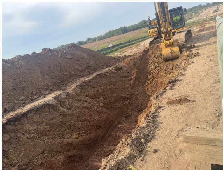
Facing north at MP 1.41, view of Otis ditching
