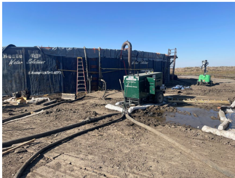
Facing northwest at Milepost 34.2, north of 165th Street, majority of water has infiltrated into the ground, contractor has lashed discharge piping to lake tank
