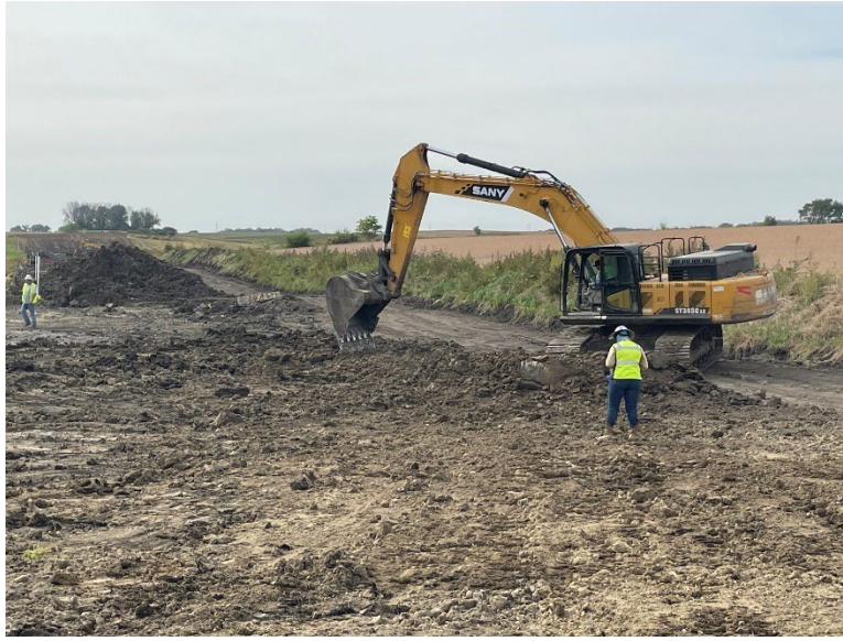
Facing southwest at MP 31.8, K&K bringing subsoil to grade south of 140th Street
